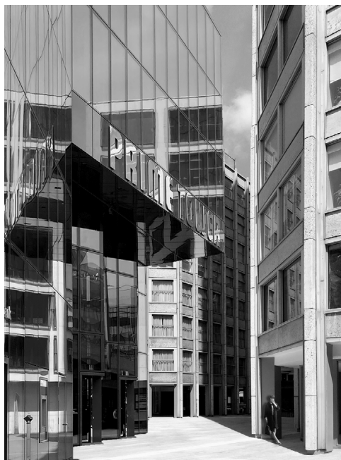
PRIMETOWER & THE ECONOMIST BUILDING A.1 | A.4 | B.1 | B.3 | C.1 | C.2 | C.4
